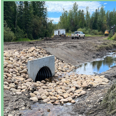
Culvert on road construction at Whitecourt Woodlands
