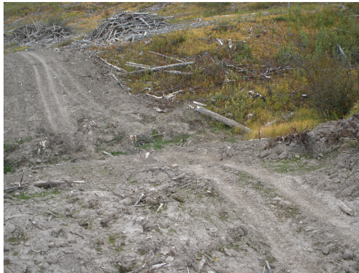
Figure 10: Example of a crossing with a 'High' Water Quality Concern Rating
