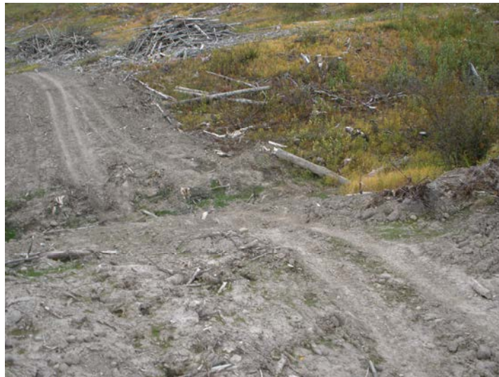
Figure 10: Example of a crossing with a ‘High’ Water Quality Concern Rating
