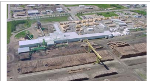
Aerial View of the Grande Prairie Sawmill Site and Log Yard
