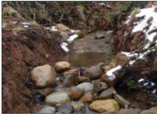
Culvert discharge armouring with rip rap.
