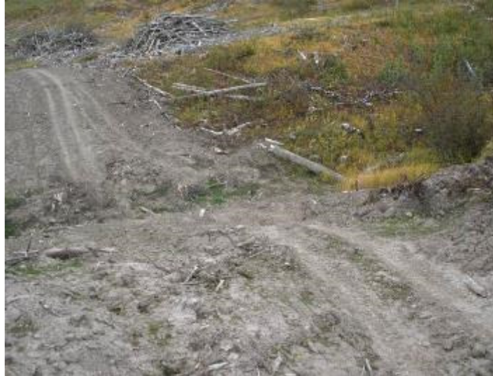
Figure 8: Example of a crossing with a ‘High’ Water Quality Concern Rating
