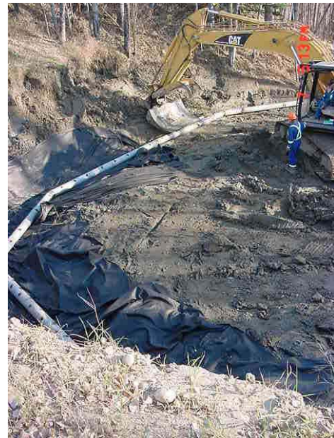
Figure 12. Remediation of Slump
