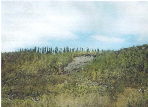
Figure 14. Minor Slump in Block W73067
