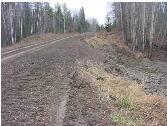
Figure 13. Remediated Slump
