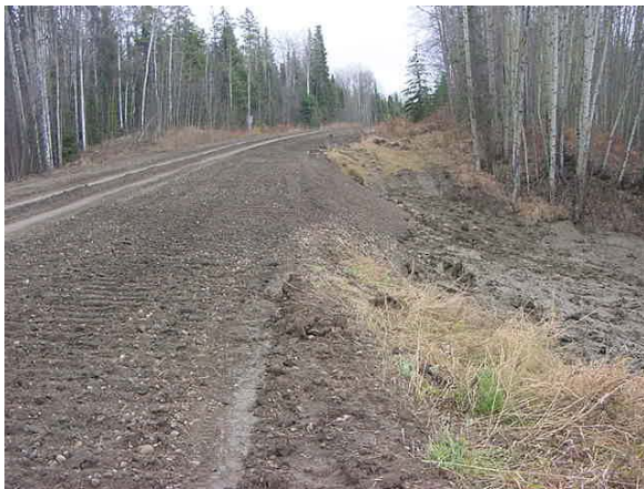
Figure 12. Remediated Slump
