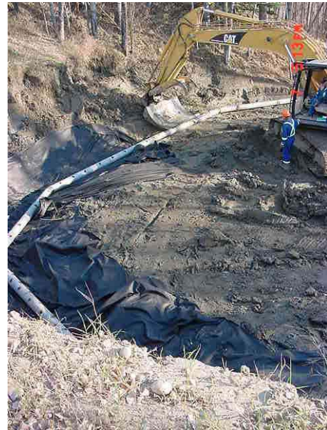
Figure 11. Remediation of Slump
