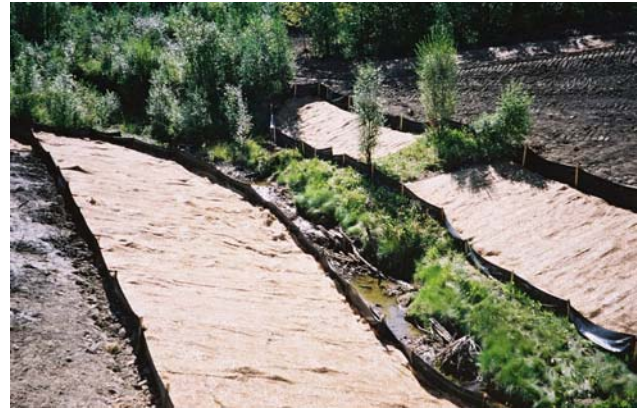
Figure 19. Use of Coco-Matting and Silt Fencing
