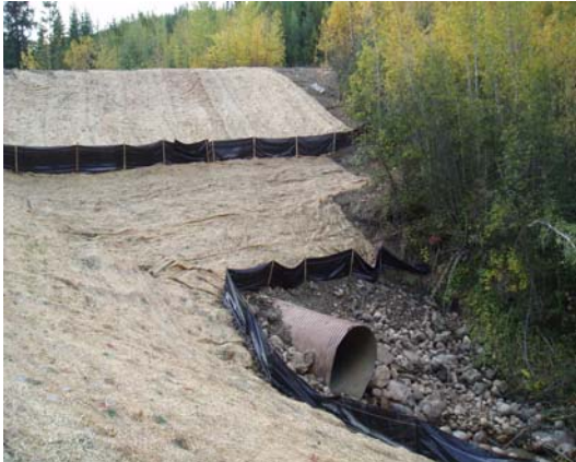
Figure 18. Use of Coco-Matting and Silt Fencing
