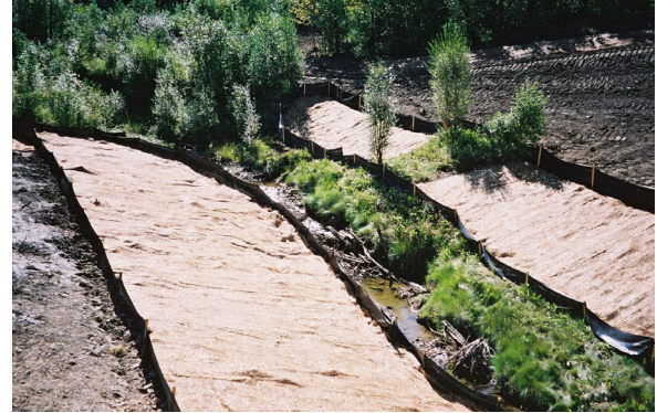
Figure 11. LOC 3735 e.g. of Geotextile
