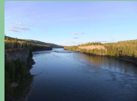
Photo of the Peace River a short distance below the W.A.C. Bennett dam. A portion of the TFL surrounds the river and reservoir. The dam represents the varied resources of the region, which as well as forestry also include extensive agriculture and oil & gas extraction.
