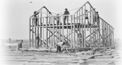
1877 Wood Frame Home
