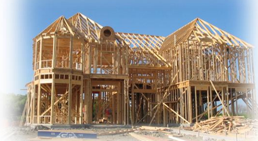
2017 Wood Frame Home
