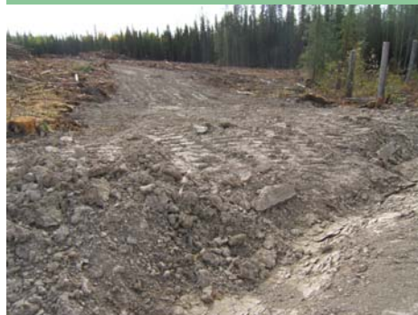
The field audit included an assessment of the full range of operational practices and activities implemented by the Participants, including the deactivation of on-block roads at the completion of harvesting.
